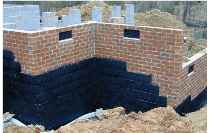
The below-grade concrete walls have damp-proof coating.
