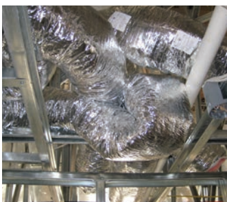
Improper Installation
