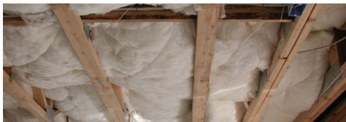
Insulation has misalignment, compression, and gaps.
