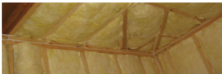
Insulation is fully aligned with air barrier with no major compressions or gaps.
